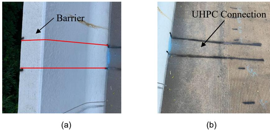
Figure 45. (a) Bridge barrier with the black spray paint lines indicating the location of the UHPC connection, transferred from underneath the deck where the UHPC is visible; and (b) marked UHPC connection region on the surface of the deck.
