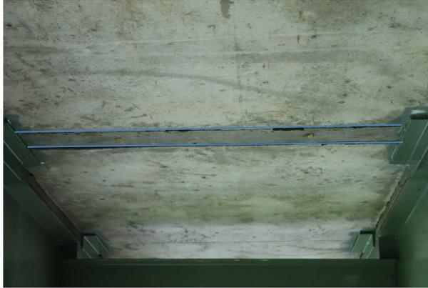
Figure 40. UHPC connection between two deck panels. Blue lines indicate UHPC connection boundaries.
