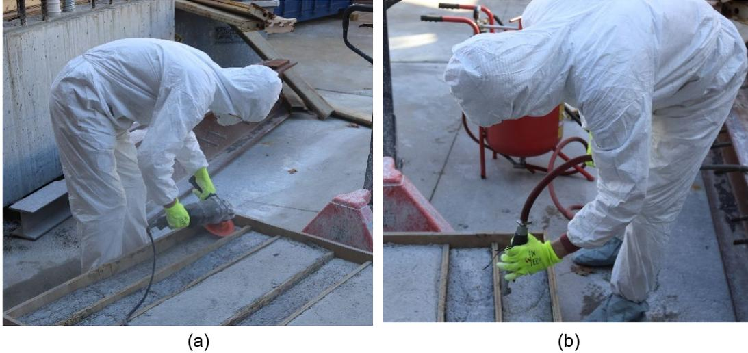
Figure 31. (a) UHPC grinding; and (b) sandblasting.
