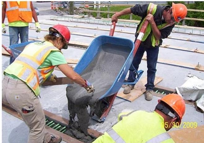
Figure 1. UHPC placement in the connection region between deck-bulb-tee girders (Graybeal, 2010).
