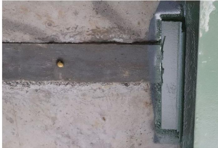
Figure 43. UHPC connection close-up.
