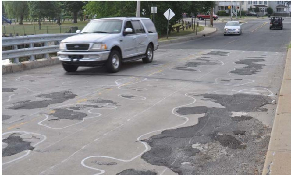
**Fig. 1.** Photo of a severely deteriorated reinforced concrete bridge deck.
