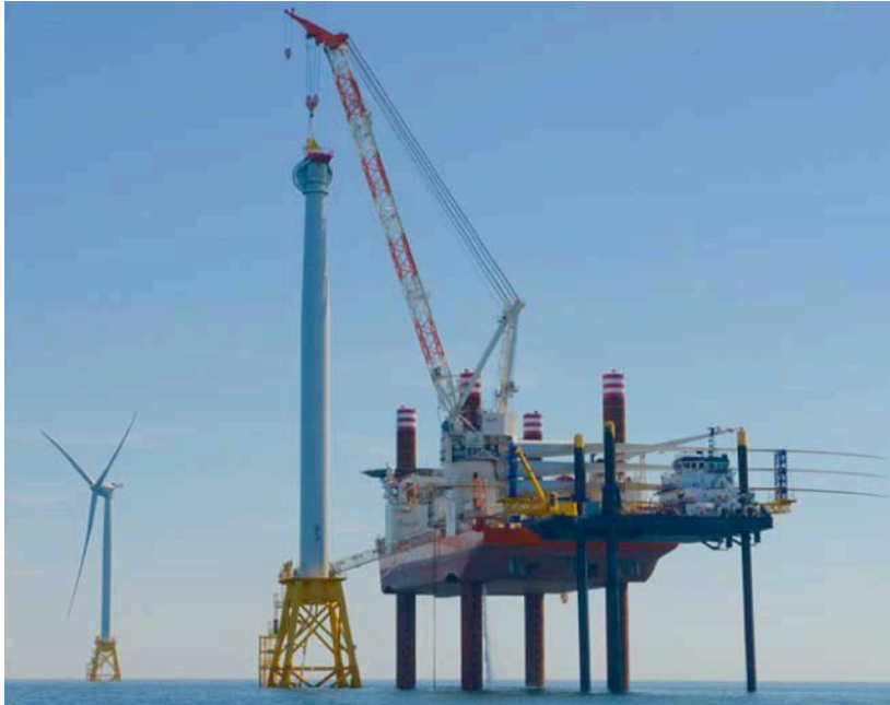
Figure 10. Traditional installation (base case): Lifting a 5 MW nacelle at Block Island, using the Brave Tern jackup vessel. From MarineLog, August 2016, © 2017 Simmons-Boardman Publishing Inc.
