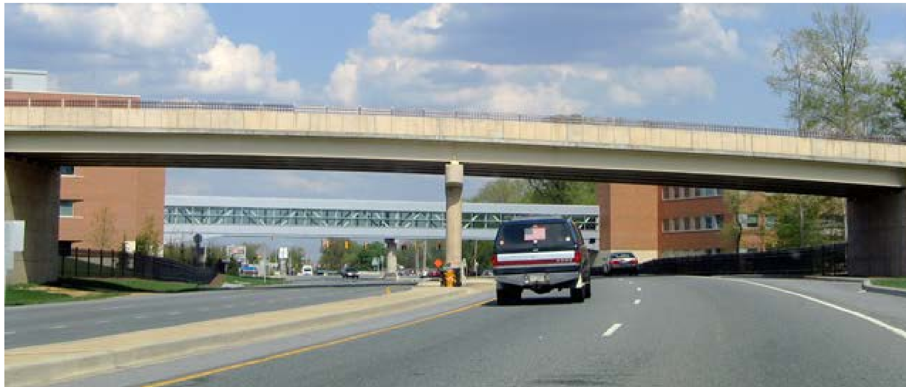
Typical highway overpass in Delaware (Source: www.aaroads.com )
