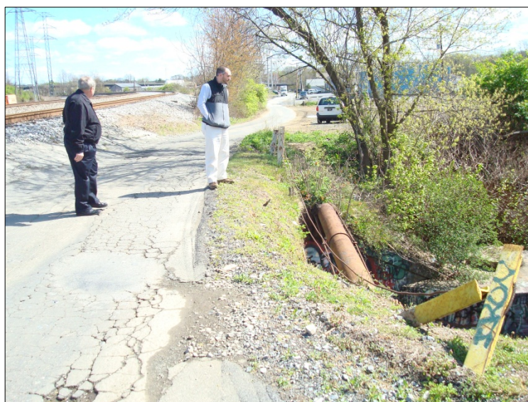
Figure 19. Poor Road Conditions and Exposed Utility Pipes at Bridge on B&O Lane
