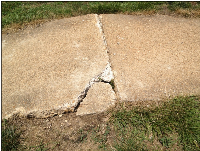
Figure 20. Broken and Uneven Sidewalk Segments
