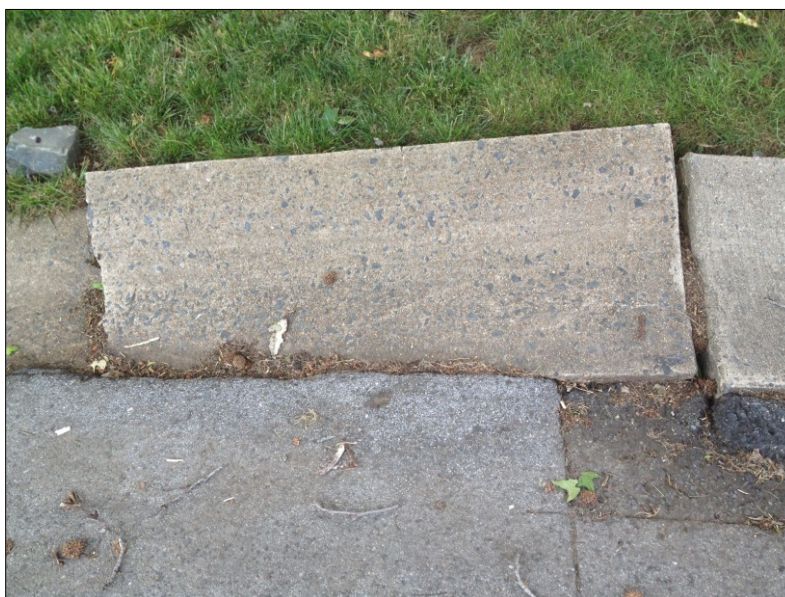
Figure 21. Dislocated Sidewalk Segments
