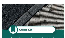
A wedge cut in an elevated curb to allow smooth passage between the sidewalk and the street.
