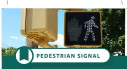
A device used at a signalized intersection with a crosswalk that informs pedestrians when to safely cross a street.
