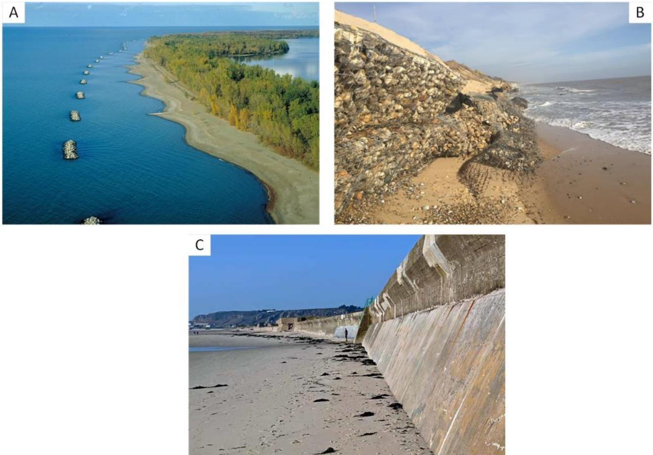
Figure 24. Examples of methods to protect beach using hard structures. A) Offshore breakwater, B) Gabion structures, C) Seawall.
