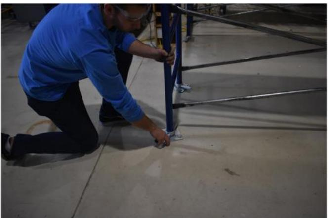
Figure A4. Pictures showing jack screw adjustment.
