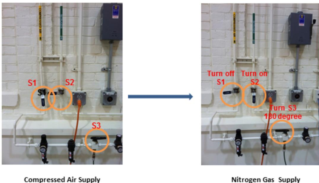
Figure 9: Switch Gas Supply from Compressed Air to Nitrogen Gas
