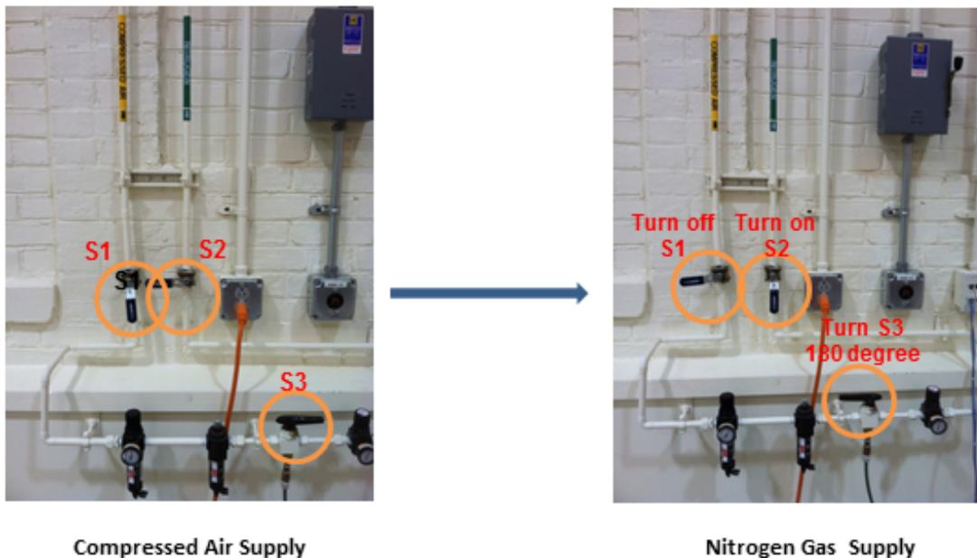
Figure 1: Switch Gas Supply from Compressed Air to Nitrogen Gas
