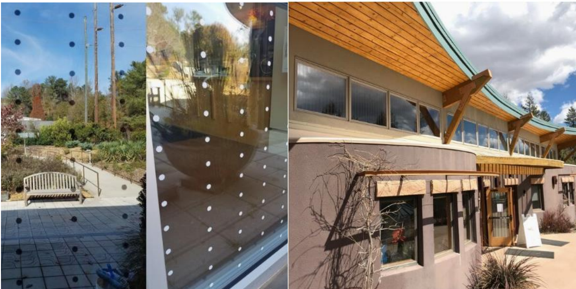
Figure 19. CollidEscape high performance bird tape applied to windows. Dot patterning (left). Stripe patterning (right). 185
