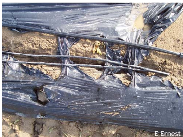
Figure 3. Split drip tape and damaged plastic (replacement tape is beside the split tape).
