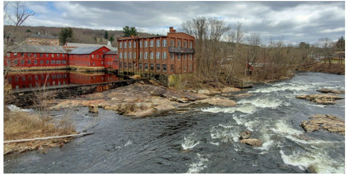
Former Collins Axe Company Factory in Collinsville, Connecticut.
