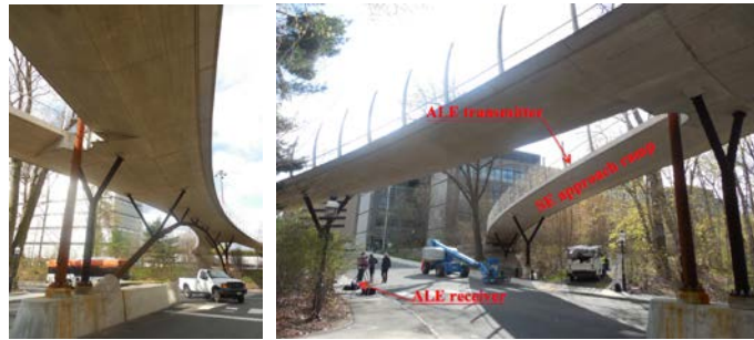
Figure 5. Strecker Bridge down-view (left) and ALE deployment (right).
