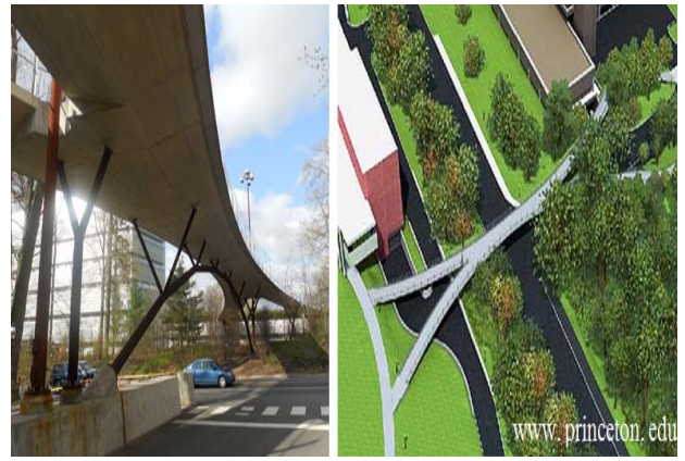
Fig. 3. Streicker Bridge at Princeton University campus (left: bottom view); (right: top view rendering – Source: www.princeton.edu)
