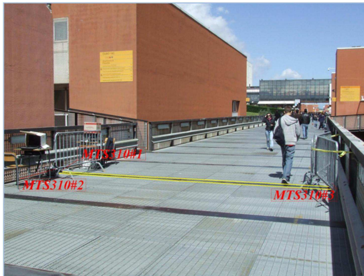
Fig.4 – Arrangement of sensors on the bridge axis
