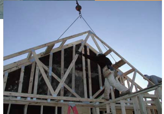
(From top): Photos 1 and 2 show unprotected workers during roof truss installation.
