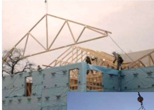
(From top): Photos 1 and 2 show unprotected workers during roof truss installation.
