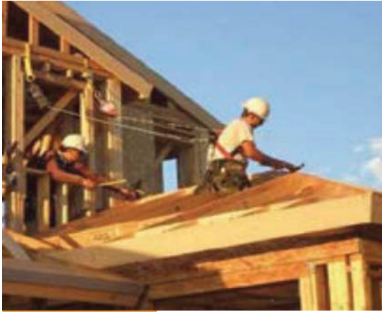
Photo 6 depicts a reusable web strap in use. This personal fall arrest anchorage was not tested in this study.
