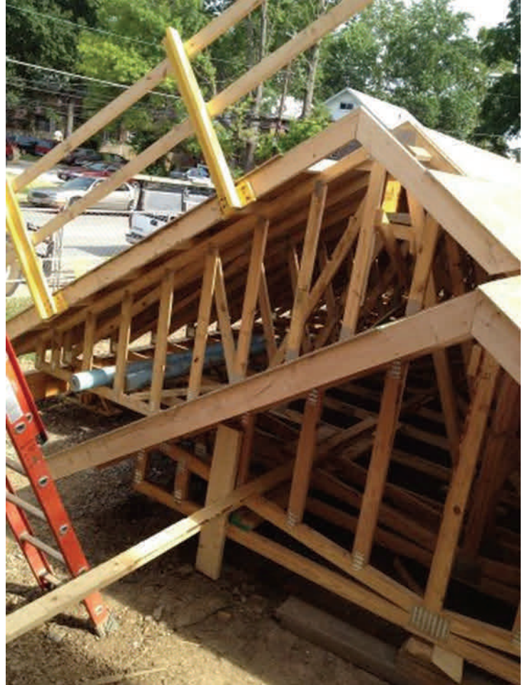
Figure 12: Guardrail on Gable End of Roof Assembly
