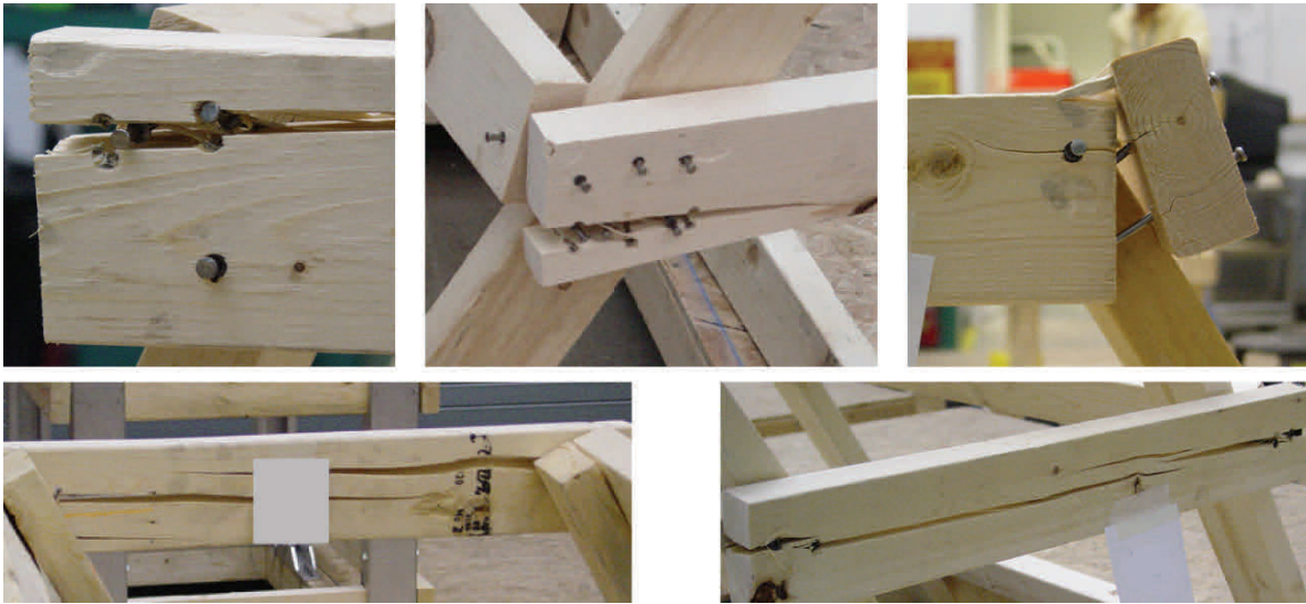
Figure 5. Examples of Wood Splitting
