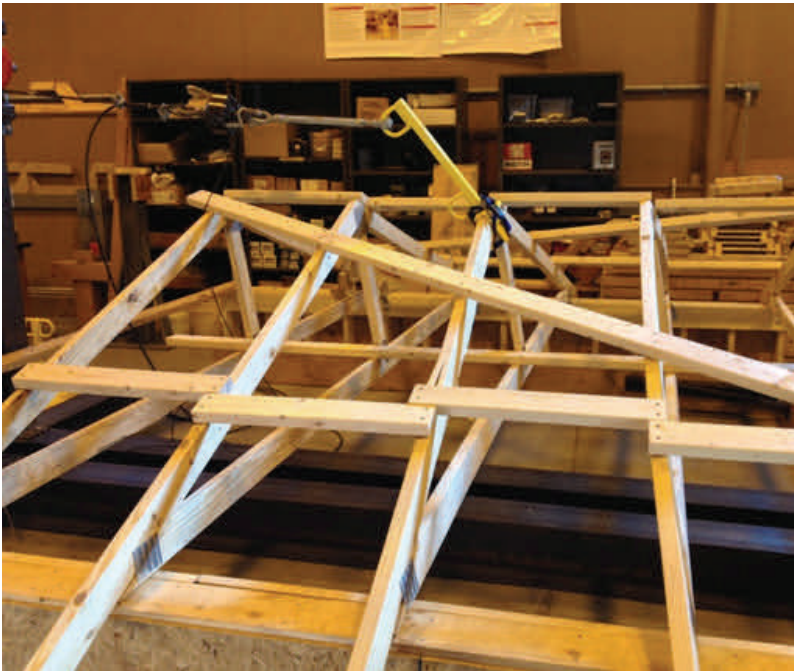
Figure 11. Loading of Five Truss System with Over the Top Bracing and Splitting of Truss
