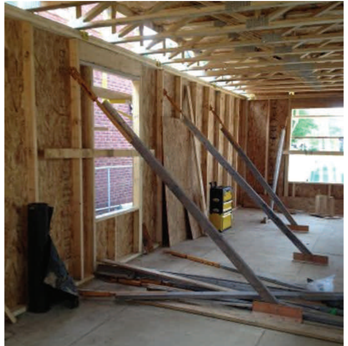
Figure 6. Bracing Required for the Scaffold System
