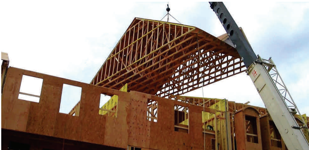
Figure 5. Lifting the Truss Assembly into Place
