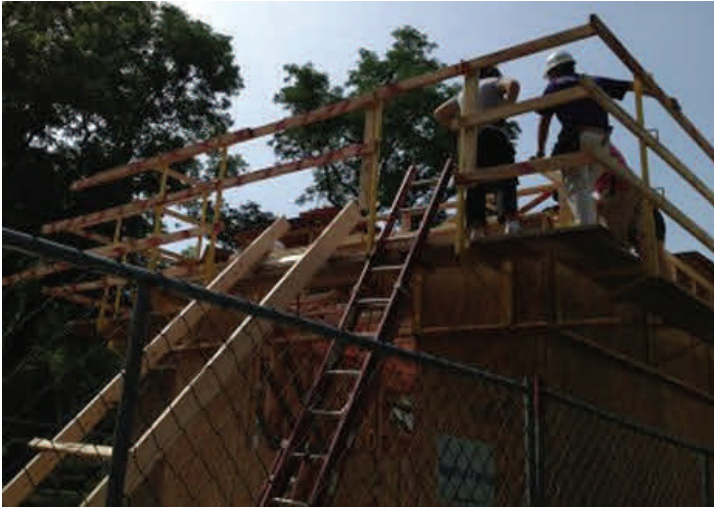
Figure 7: Three Rows of Guardrail on Hanging Scaffold
