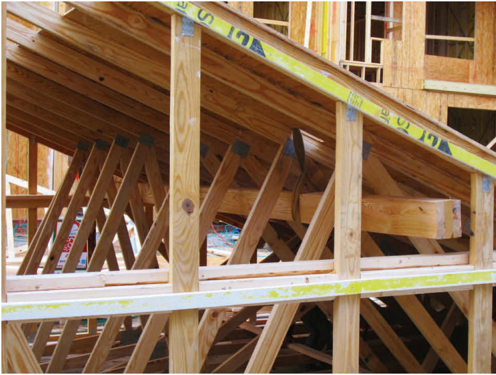
Figure 4. Lifting Beam Placement within the Truss Raft Structure
