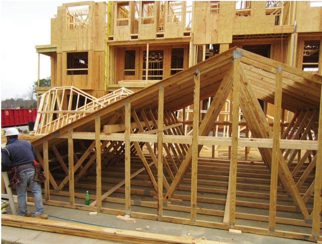
Figure 2. Bracing and Sheathing Installed
