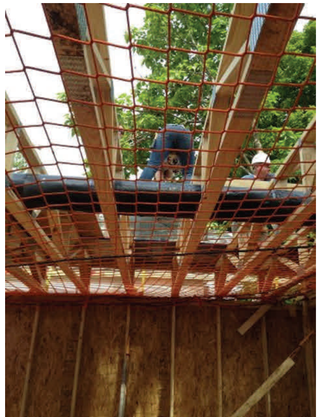
Figure 1. Net Under Floor Joists on 2 Foot Centers
