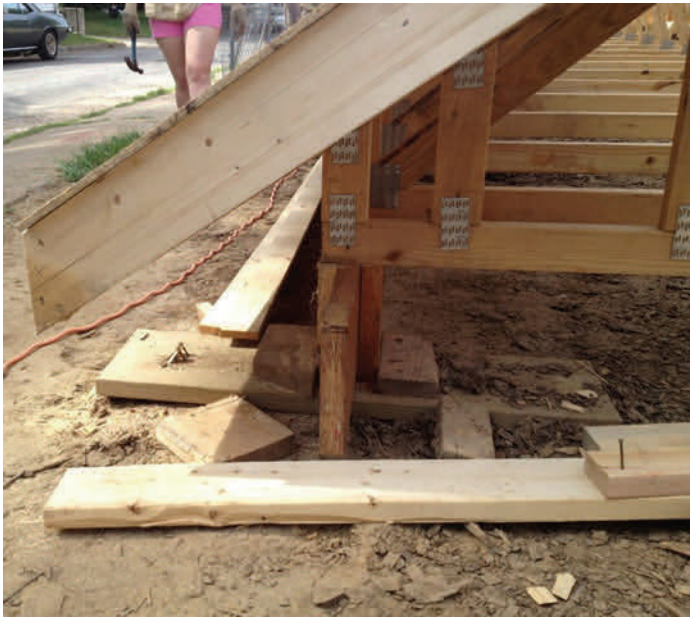
Figure 11: Stationary Base for Roof Assembly
