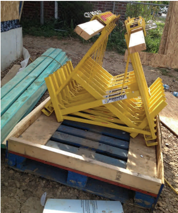
Figure 8: Storage Bin for Hanging Scaffold
