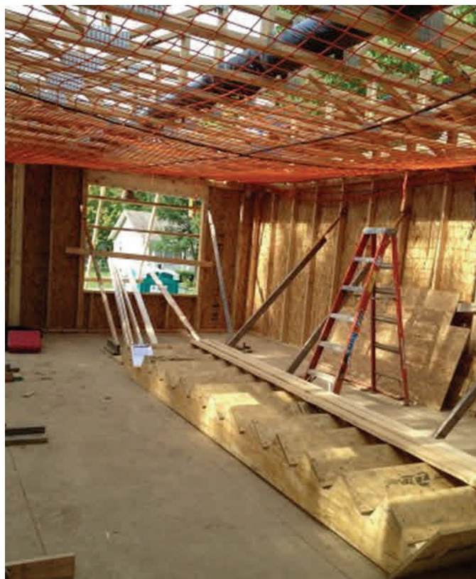
Figure 3. Net Pulled Snugly in Place
