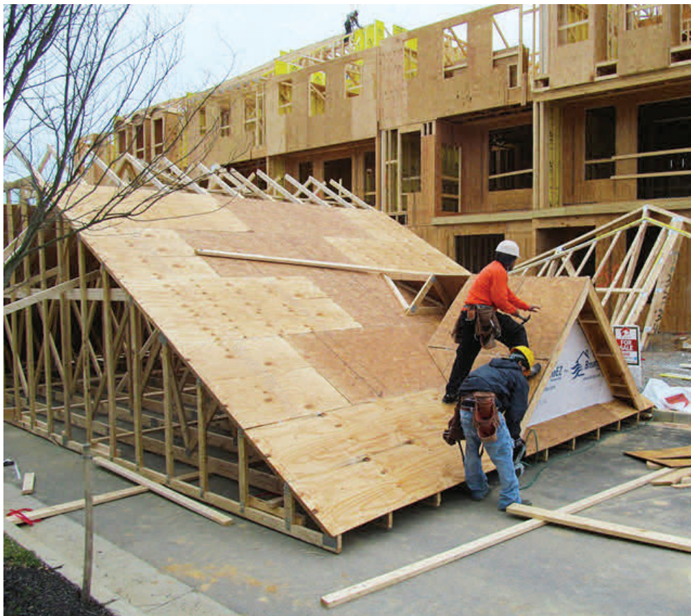
Figure 3. Trusses, Sheathing, and Front Gable Installed
