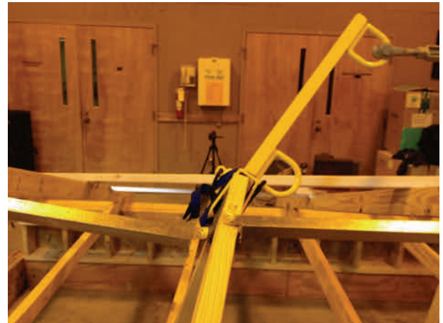
Figure 12. Metal Engineered Bracing Pulled From Truss After Failure
