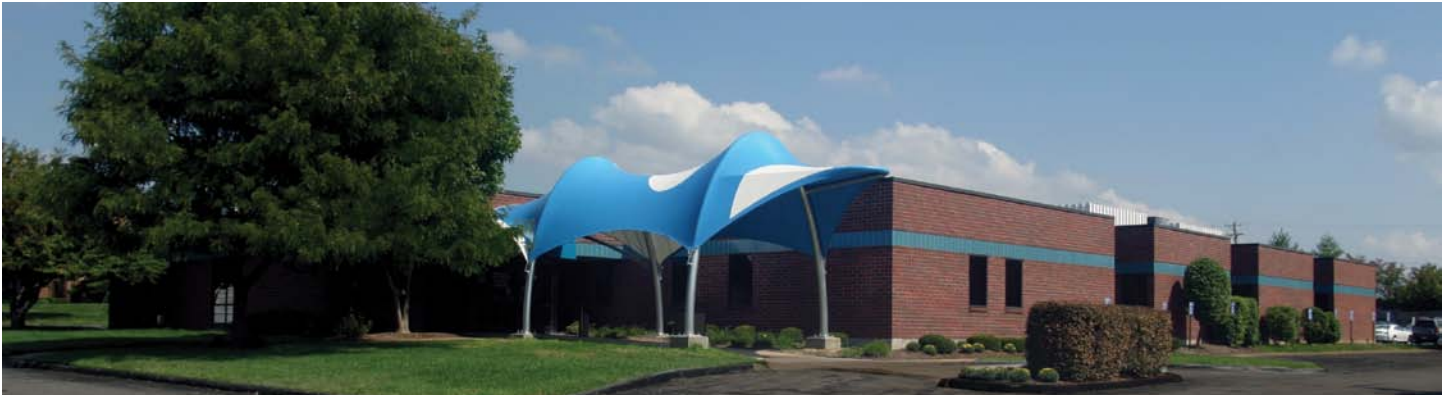
People's Health Centers North County Facility.
