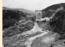
The dam was designed and built between 1924 and 1926 by the Los Angeles Department of Water and Power. When the dam catastrophically fails, the resulting flood takes the lives of an estimated 431 people.<sup>10</sup>
