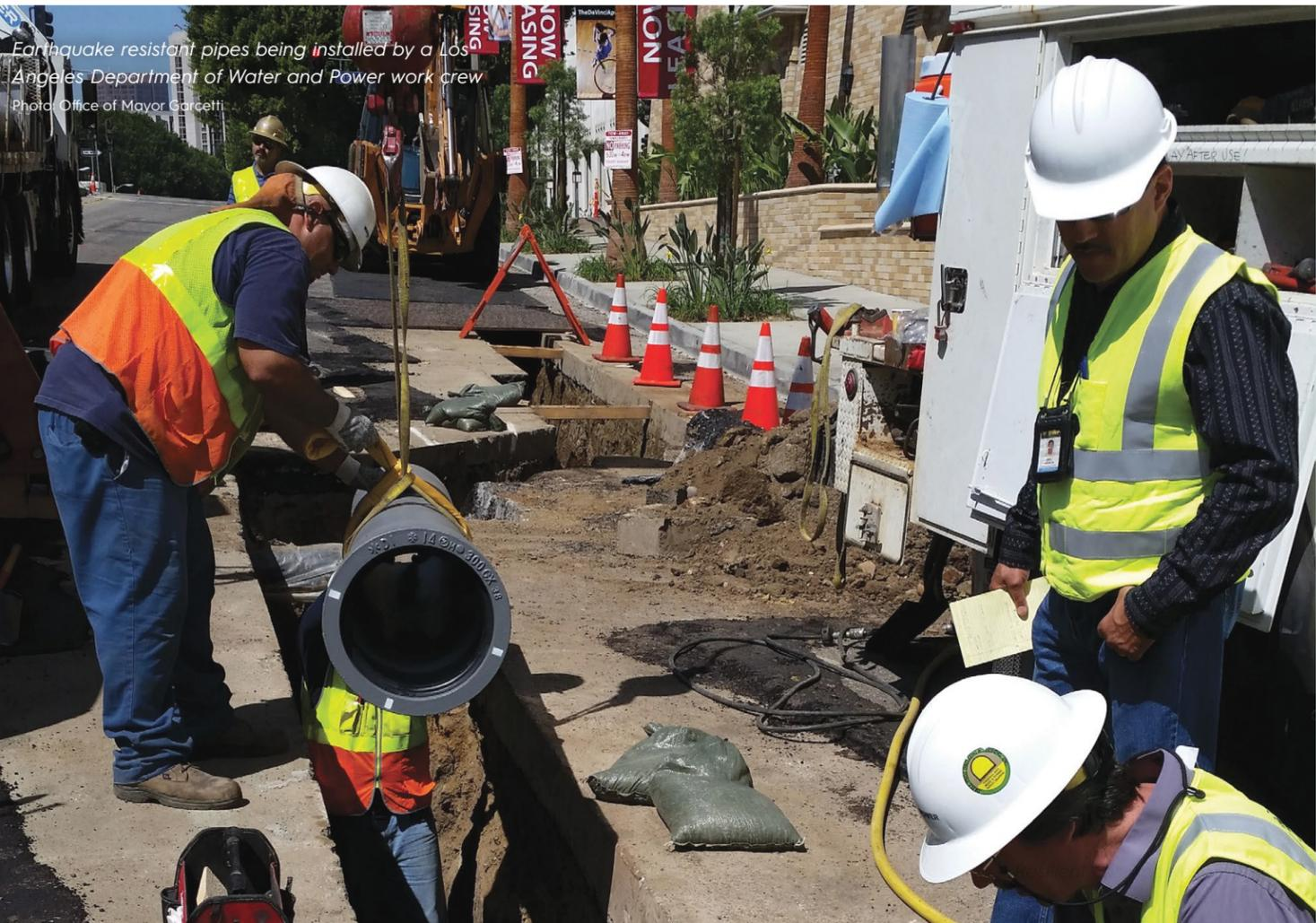
Earthquake resistant pipes being installed by a Los Angeles Department of Water and Power work crew
