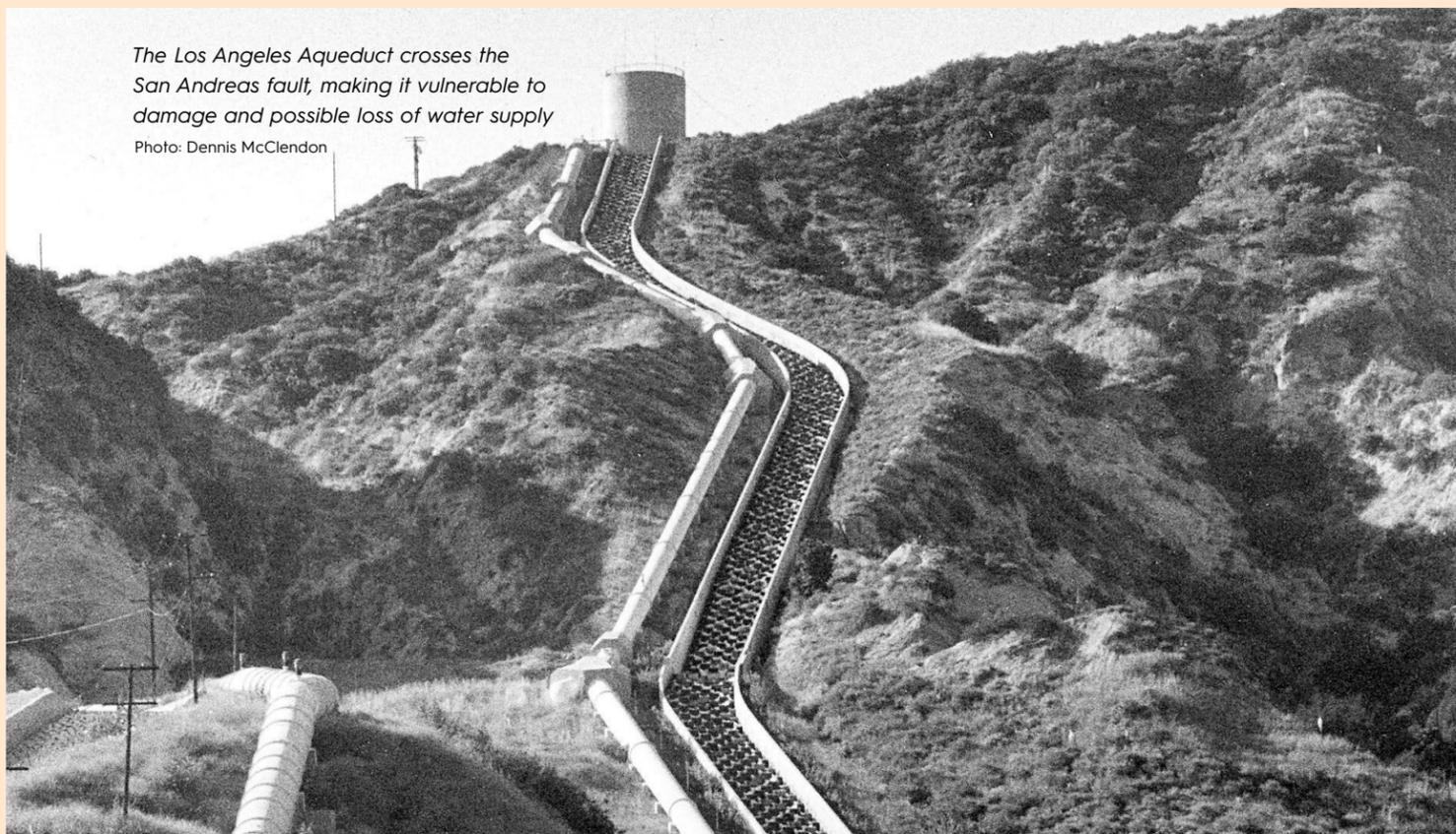
*The Los Angeles Aqueduct crosses the San Andreas fault, making it vulnerable to damage and possible loss of water supply*
