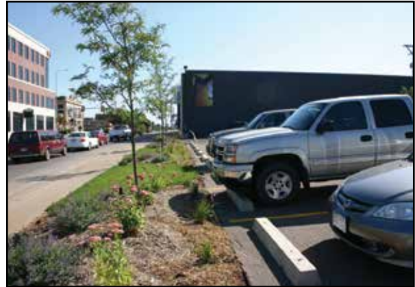
After street landscape buffer was installed.
