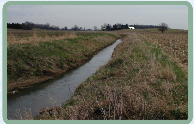
Figure 2. A headwater channel that has been straightened and deepened to a trapezoidal geometry.
