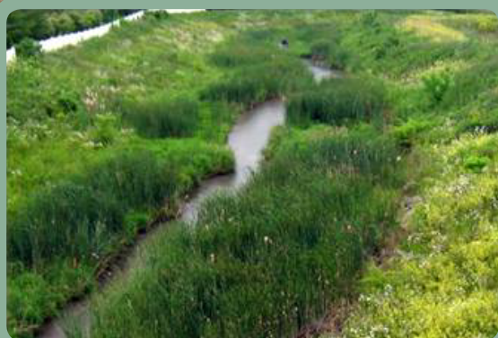
Figure 6. A self-forming channel just after construction (above); the same channel three growing seasons after construction (right).
