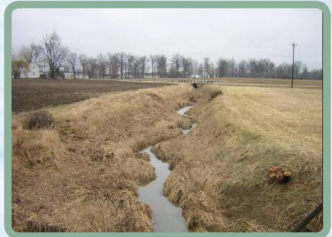
Figure 4. In an existing modified channel system, nature has formed a meandering inset channel and attached floodplain (benches).
