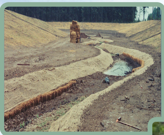
Figure 7. Constructing a channel and floodplain (above); the channel immediately after construction (right).
