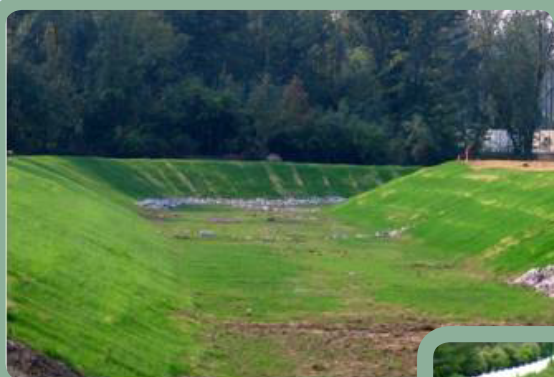
Figure 6. A self-forming channel just after construction (above); the same channel three growing seasons after construction (right).
