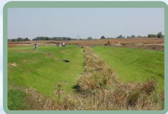
Figure 8. Construction of a two-stage ditch. The benches were made wide enough for vehicle access (top) and are located just below subsurface drainage outlets (above). Discharge from the outlets flows across vegetated benches.
