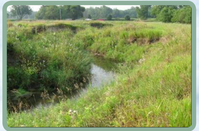
Figure 3. Bank instability in a ditch.
