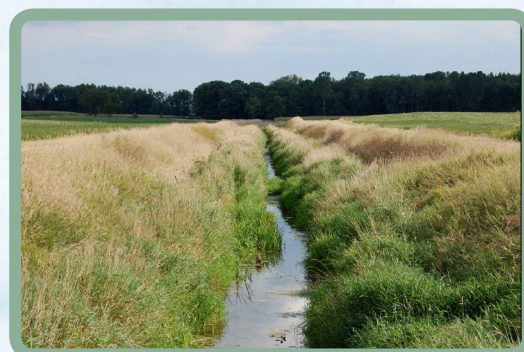
Figure 1. A two-stage channel system 6 years after construction.
