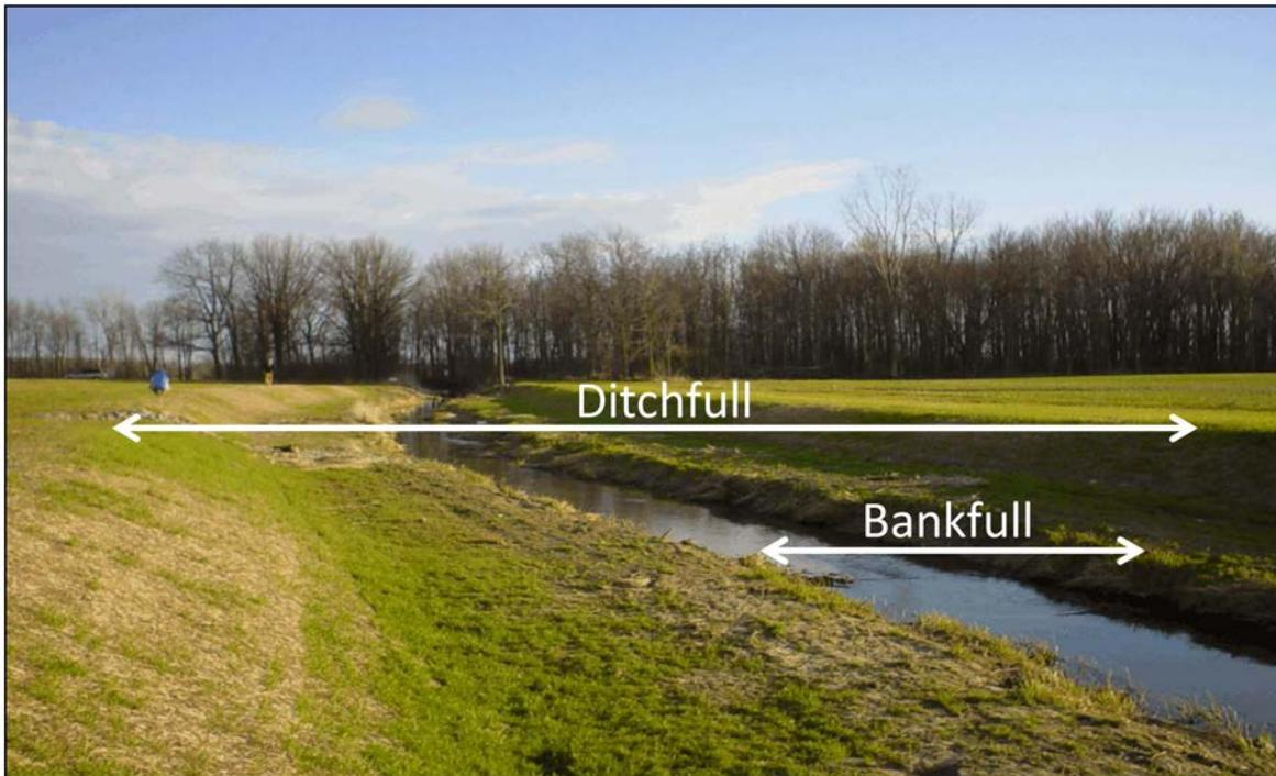
Figure 8. Diagram of ditchfull and bankfull locations on a two-stage ditch.
