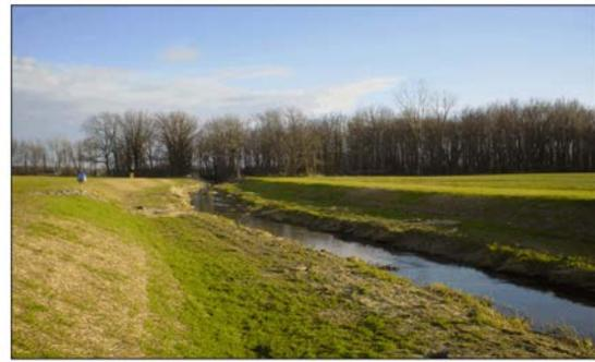
Figure 2. A two-stage ditch.
