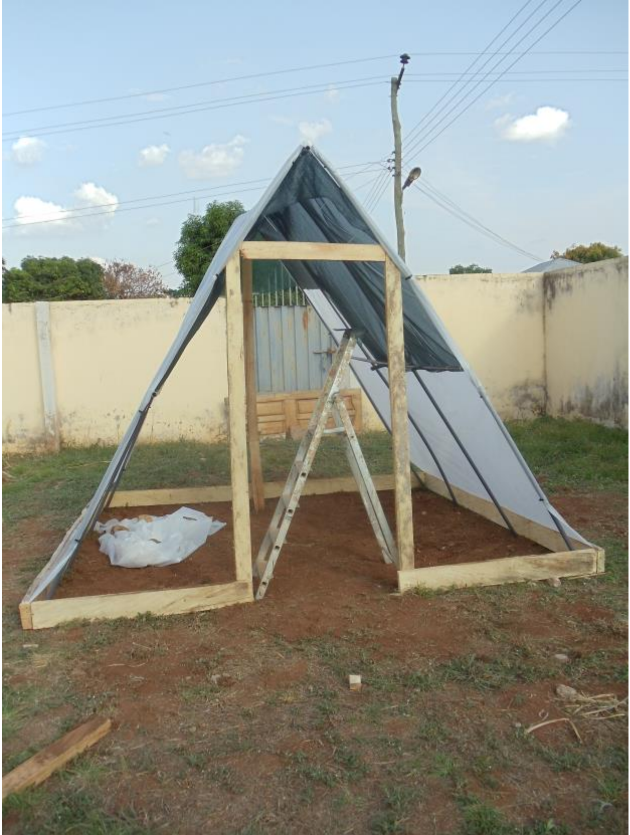
Figure 2: Construction completed after day 3.
