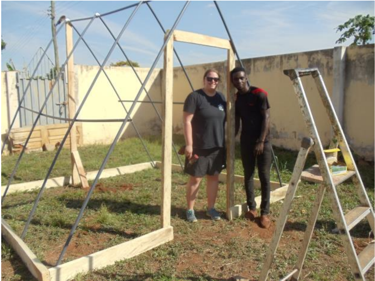
Figure 1: Construction completed after work day 2.
