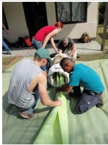
Using an old bucket to enclose the end of the biodigester.
