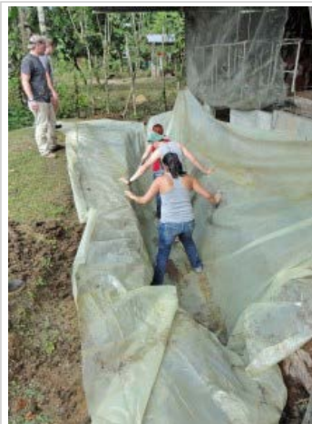
Cleaning out the hole where the new biodigester will go. An old one was there previously.
