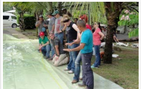
Starting the biodigester project. The biodigester is made mainly of a thick sheet of plastic looped around and closed off at the ends.
