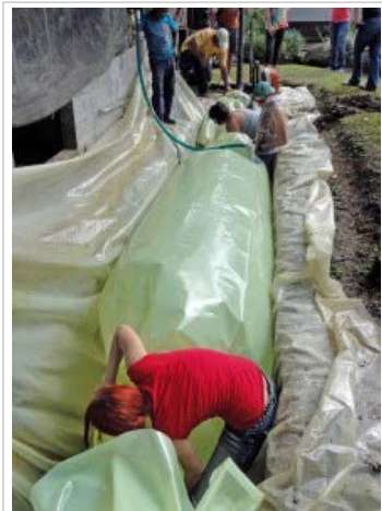
Filling the new biodigester with air.
