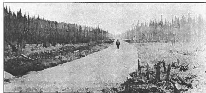
The roadbed for a new railway, circa 1900–1905. (Library of Congress)
