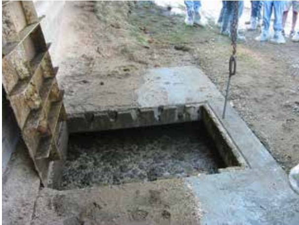
Figure 8.1 A manure pit is a confined space work area. Many lives have been lost in manure pits due to toxic gases and lack of oxygen. Credit: PSU Ag Safety.
