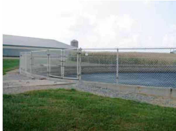
Figure 8.13 Open manure storage areas pose a less deadly gas hazard than belowground pits. The major hazard of the open manure storage is drowning. Fencing and warning signs alert people to the liquid manure hazard. Credit: J. Mathison.
