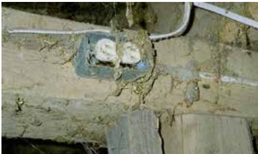
Figure 5.33 Dusty, dirty conditions in agriculture contribute to increased fire hazards. What materials in this picture are considered Class A fuel sources? Credit: PSU Ag Safety.
