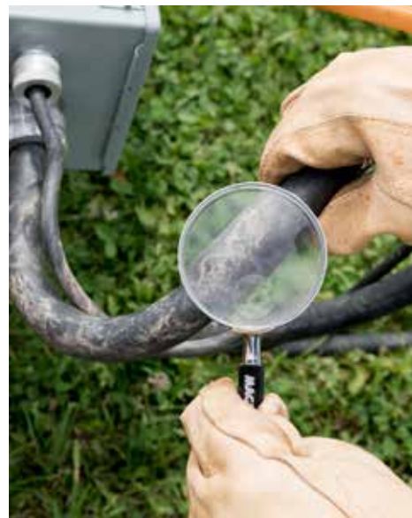
Figure 3.28 Use a magnifying glass, mirror, or piece of cardboard to check for high-pressure hydraulic leaks. Do not use your hand! Pinhole leaks are often invisible. Credit: J. Mathison.
