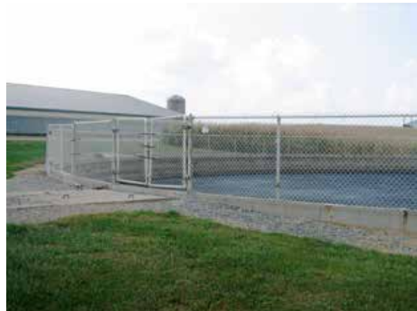
Figure 8.13 Open manure storage areas pose a less deadly gas hazard than belowground pits. The major hazard of the open manure storage is drowning. Fencing and warning signs alert people to the liquid manure hazard. Credit: J. Mathison.
