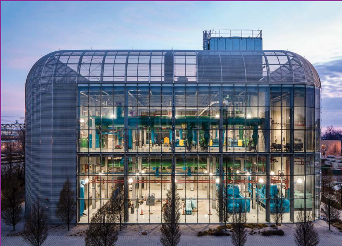
The Environmental Frontiers program focuses on sustainability at the University of Chicago campus, including water use from the South Campus Chiller Plant, pictured.
