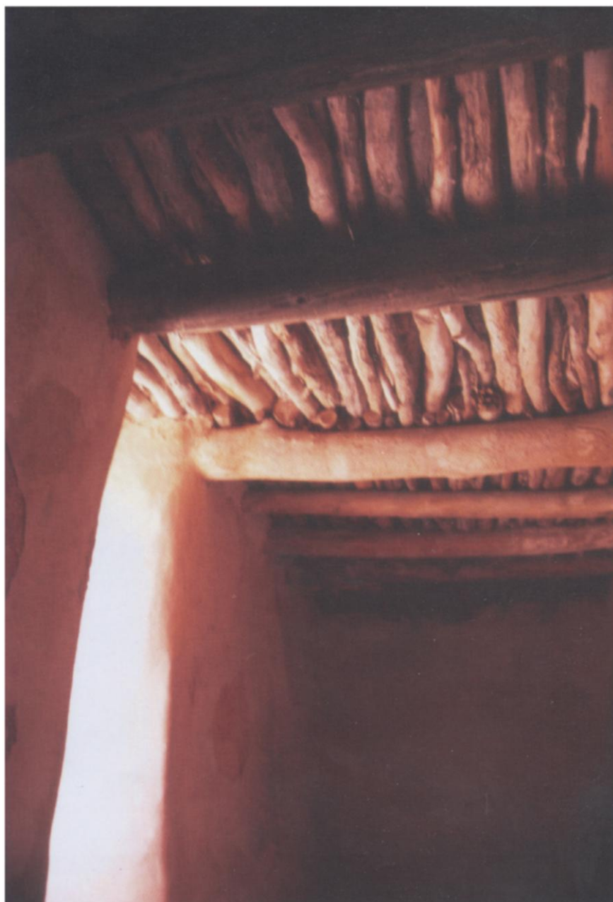
A reconstructed wooden ceiling of a four-room house at Tel Qasile. Twenty-seven tons of wood would have been required to support both floors of the house at Tall al-'Umayri!
