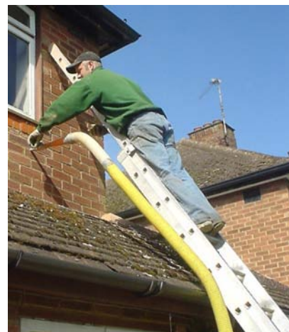
Figure 21.5. Cavity-wall insulation going in.
