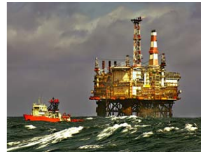
Figure 10.4. The Magnus platform in the northern UK sector of the North Sea contains 71 000 tons of steel. In the year 2000 this platform delivered 3.8 million tons of oil and gas – a power of 5 GW. The platform cost £1.1 billion.
