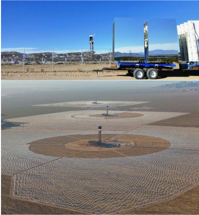
Figure 12.2: Top: Heliostat mirrors being delivered to the Ivanpah Solar Electric Generating System in Nevada ( Wikimedia Commons ). Bottom: aerial view of the full facility nearing its 2014 completion. it has 173,500 heliostats and 392 MW capacity ( Brightsource Energy ).
