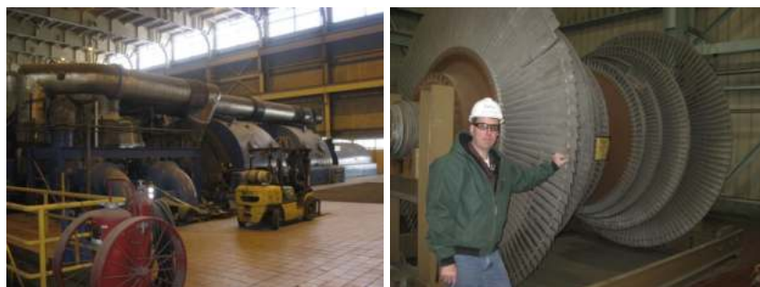
Figure 9.3: At left: the turbines and generator (rearmost cylinder) for one of the coal units at the Eddystone Generating Station just south of the Philadelphia airport. At right, plant manager Bryan Bennett of Exelon stands in front of a fan that has been removed from one of the turbines. The plant, built in the 1960's, has since been decommissioned. Photos by Gary Bernstein.
