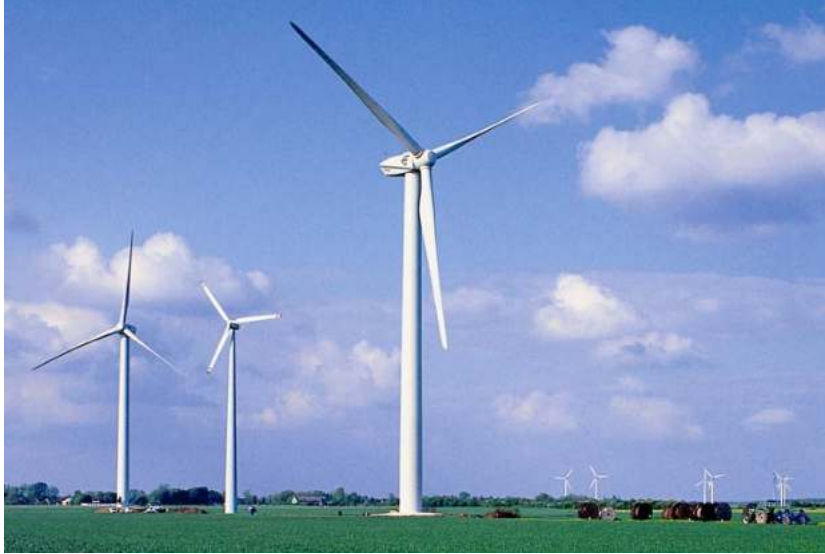
Figure 10.2: 5 MW wind turbines with 126-m rotor diameter. Each blade is about as long as the wingspan of a Boeing 747. This is built by Repower and installed in Germany. note the tractor at lower right for scale. Source .
