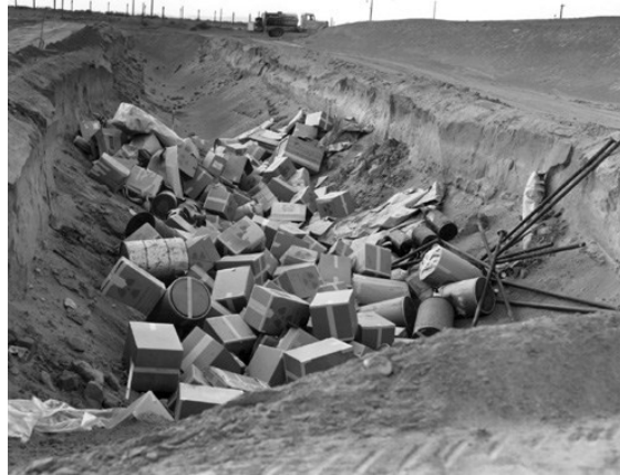
Figure 5: Transuranic waste in a trench at the Hanford Reservation in the 1950s. The trenches would be covered with dirt and the soil and groundwater would be contaminated.
