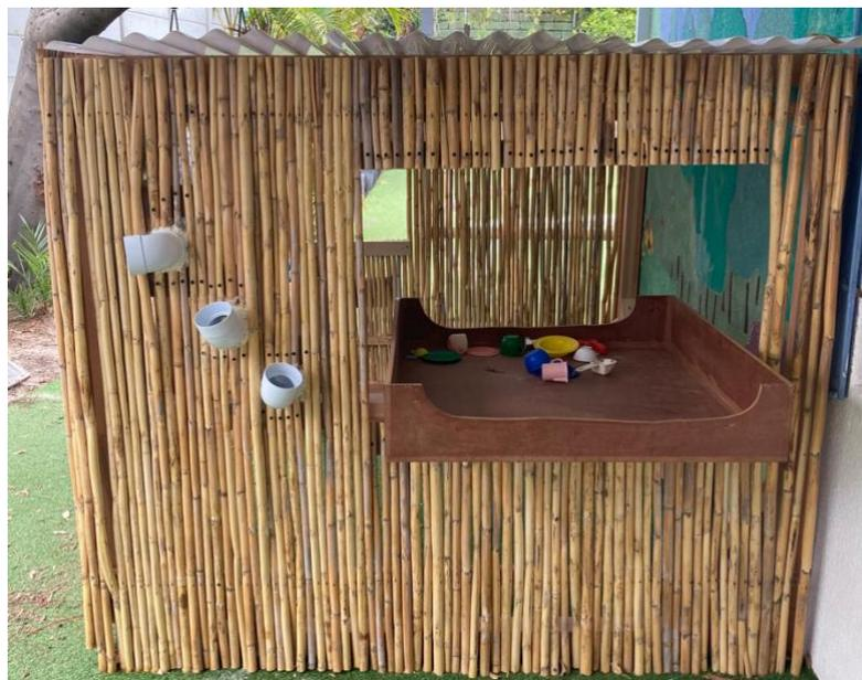
*Figure 27: Picture of Bamboo Siding*
