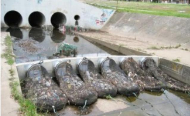
Figure 6: StormX Netting Trash Trap in use (Image Credit: StormX, 2020)
