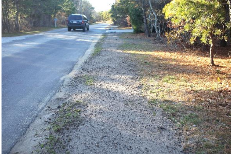
Figure 4.20: Filled easement trench on Skyline Drive
