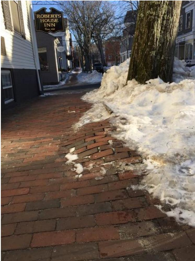
**Figure 2.3 Example of Tree Roots Damaging the Brick Sidewalk**
