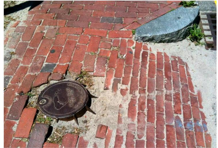
**Figure 2.4 Example of Uneven Footing**
