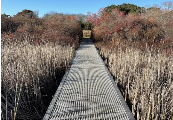
Figure 31: Gardner Farm Wetland Bridge (NLB)
