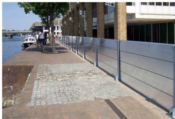
Figure 44: Example of a multi-panel flood barrier system with modular components (floodbarrier.com).
