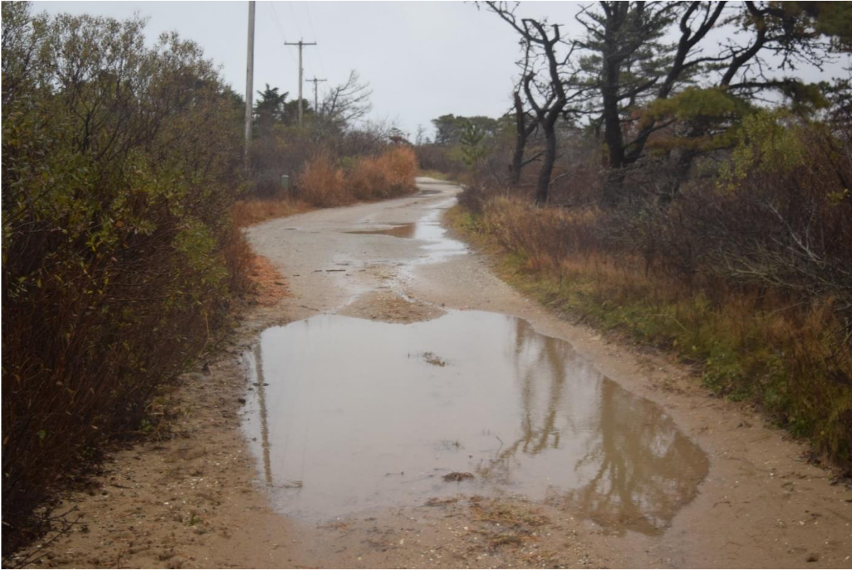
Picture of Eel Point Road after rainfall.
