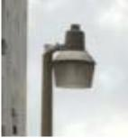
Improper Shielding: Shield fully encompasses the bulb but does not prevent light from • traveling above the horizontal due to the angle
