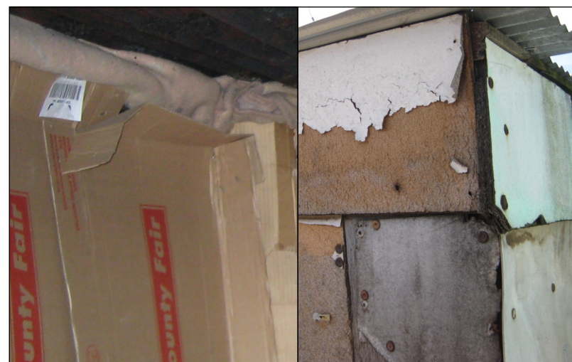
Figure 5-8: Current shack insulation methods include cardboard on walls, newspaper and other random materials in gaps and boards on the exterior.
