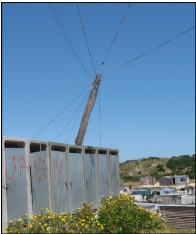
Figure 5-4: Those with informal connections must put up their own wires and poles.
