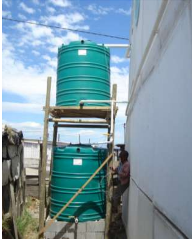
Figure 32: PVC Connecting the Storage Tanks
