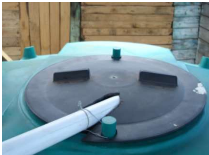
Figure 33: Cover of Overflow Tank
