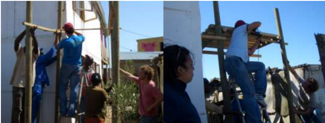
Figure 25: Installing the Tank Stands
