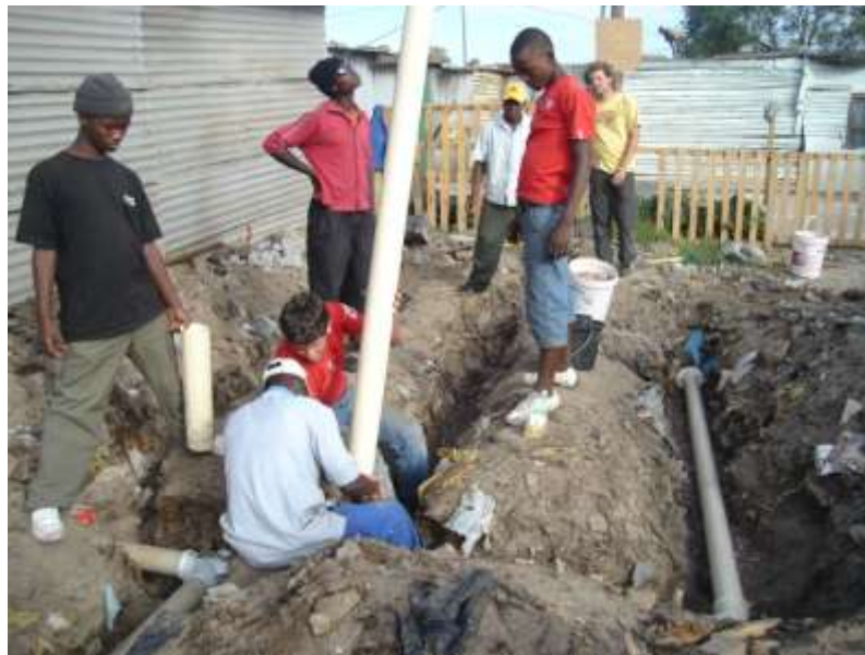
Figure 40: Installing the Soakaway System
