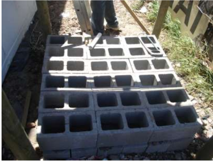
Figure 26: Raised Platform for Lower Tanks
