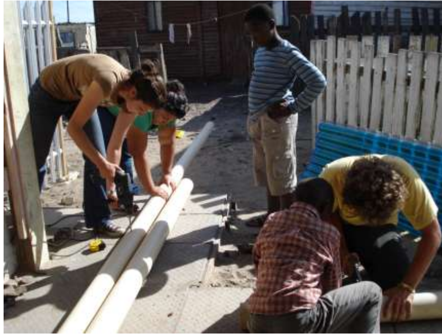
Figure 38: Drilling Holes in the Irrigation Pipe
