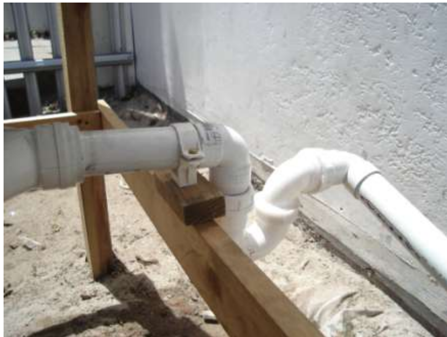
Figure 37: Trap Configuration
