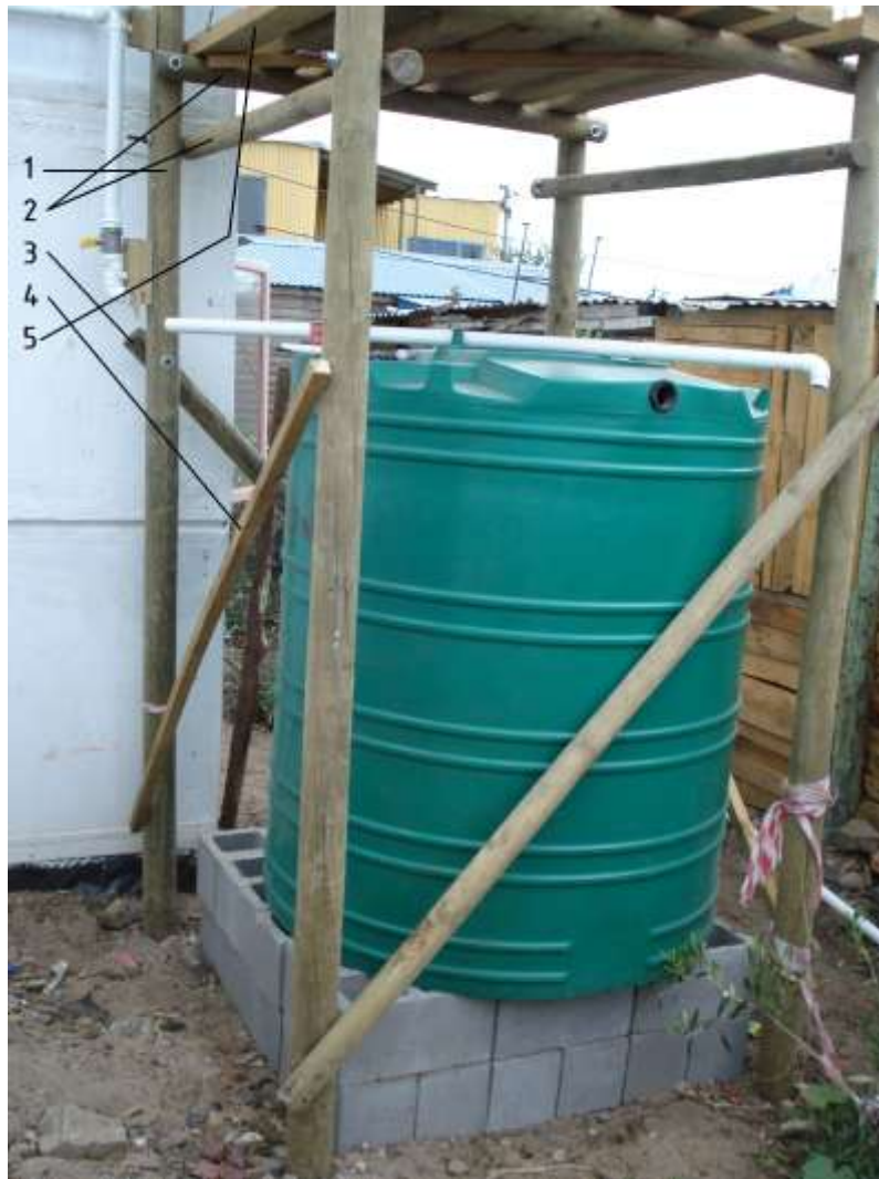
Figure 24: Tank Stand Components
