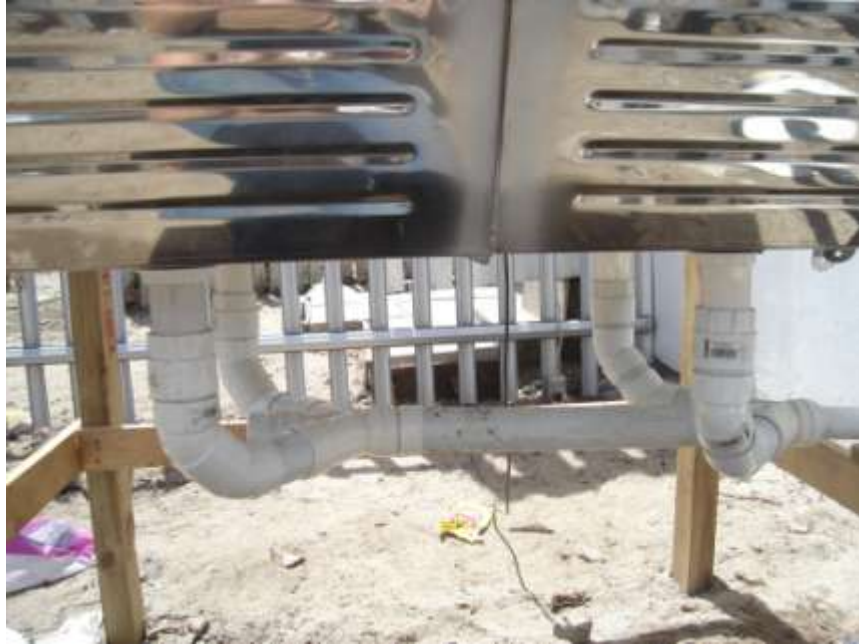
Figure 36: Drainage Configuration
