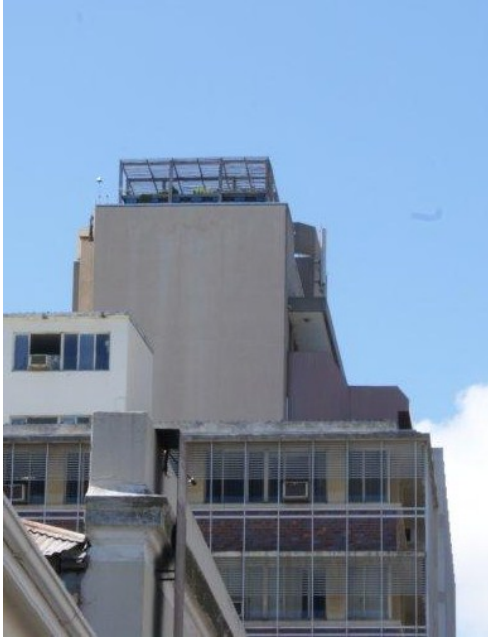
Figure 2: Street level view of the 44 Wale Street rooftop garden
