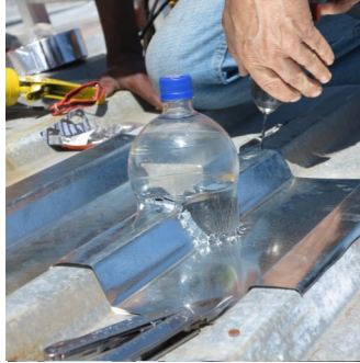
Drill Holes for Rivets
