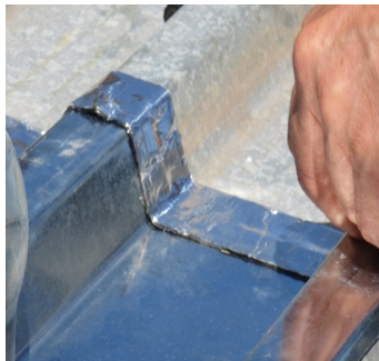
Apply Flashband at top
