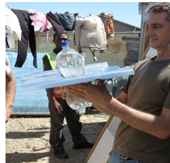
Carefully test bottle fits
