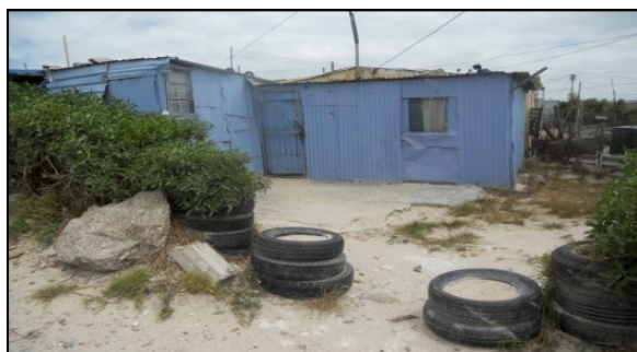
Figure 5: Stacked tyres filled with sand
