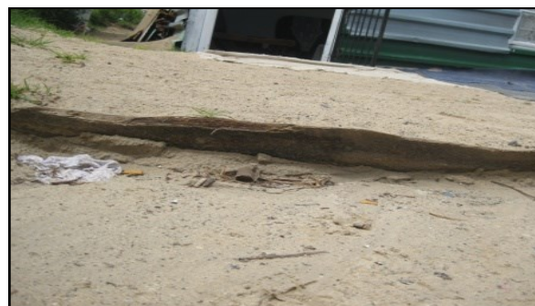
Figure 12: Wooden ledge preventing water flow into a home
