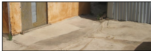
Figure 11: Boards used to create a ramp leading to the doorway of a shack
