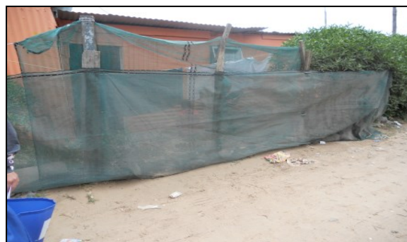
Figure 4: Double-layer shadecloth fence against an informal settlement shack
