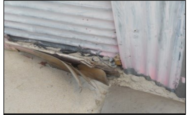
Figure 14: Thick plastic placed between the walls of a shack
