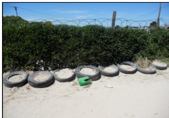
Figure 6: Wall of half-buried tyres
