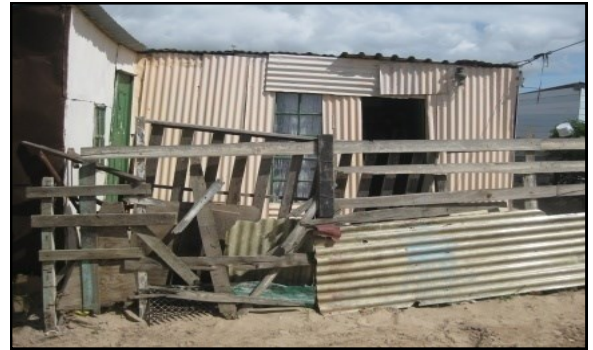
Figure 2: Improvised fence of wooden boards and metal sheeting
