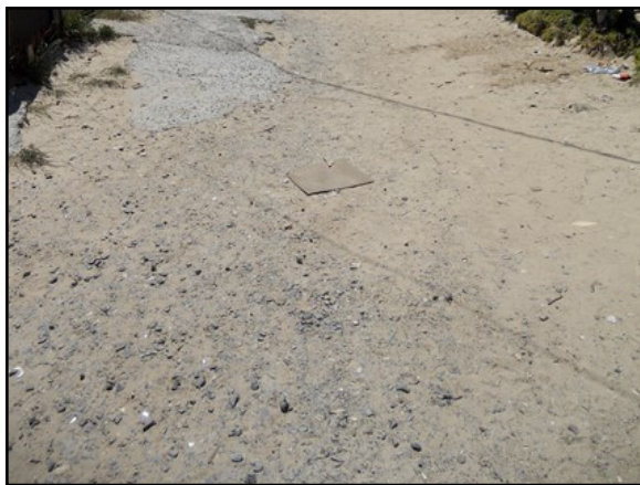
Figure 16: Small and medium-sized rocks embedded in a road
