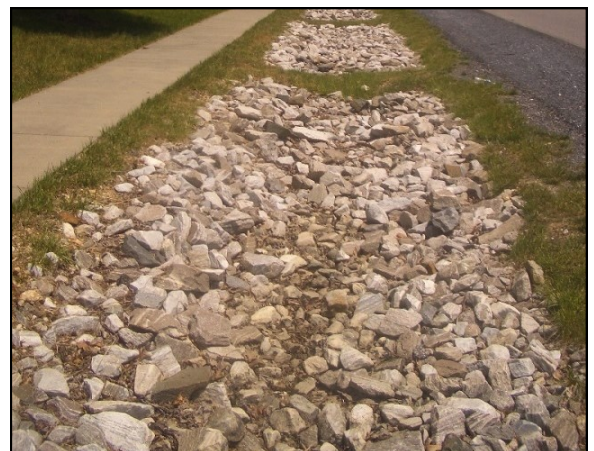
Figure 14: Rock-filled trench that encourages water to sink into the soil (Infiltration Trenches, 2007)
