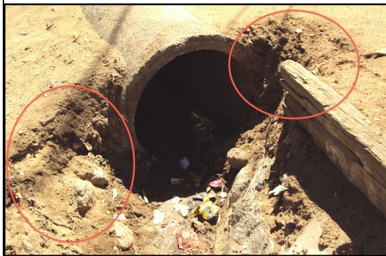
Figure 24: Bank erosion along a greywater channel in Langrug, South Africa
