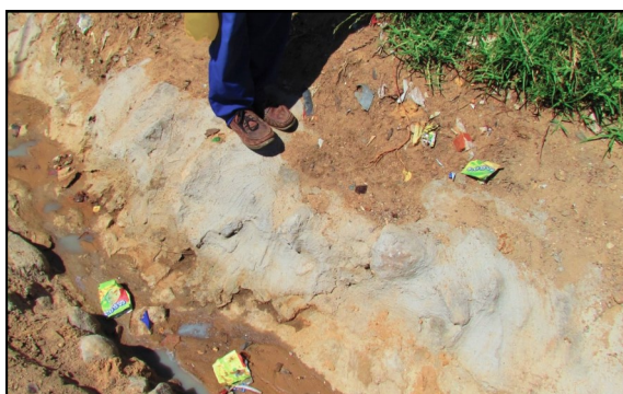
Figure 28: Cement channel base extended up the channel walls to prevent erosion
