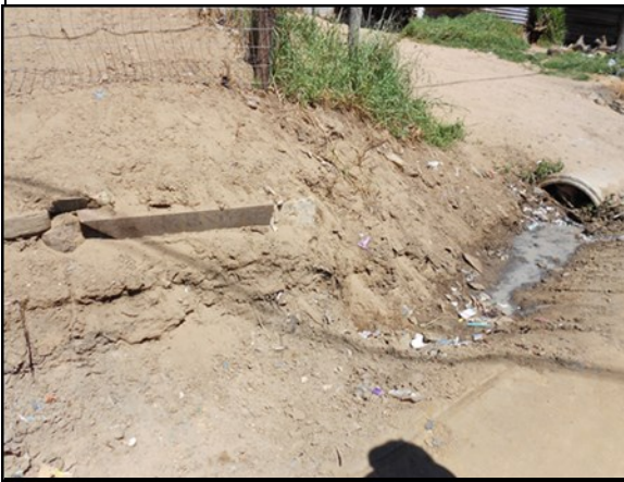
Figure 23: A clogged greywater channel in Langrug, South Africa
