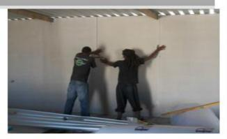
The drywall cleans gives a nice clean finish on the inside. It is also critical to have some ventilation so the room does not get hot and stuffy. Vents can be added in the front and back. By drilling holes and through the frame walls and placing a small vent on both the inside and the outside. This is a safe way to ensure they are not stolen while still providing air flow.
